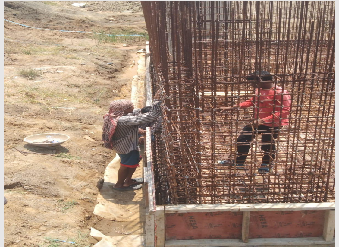
UG Sump shuttering work in progress.
