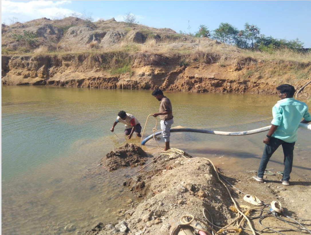
Dewatering work in progress
