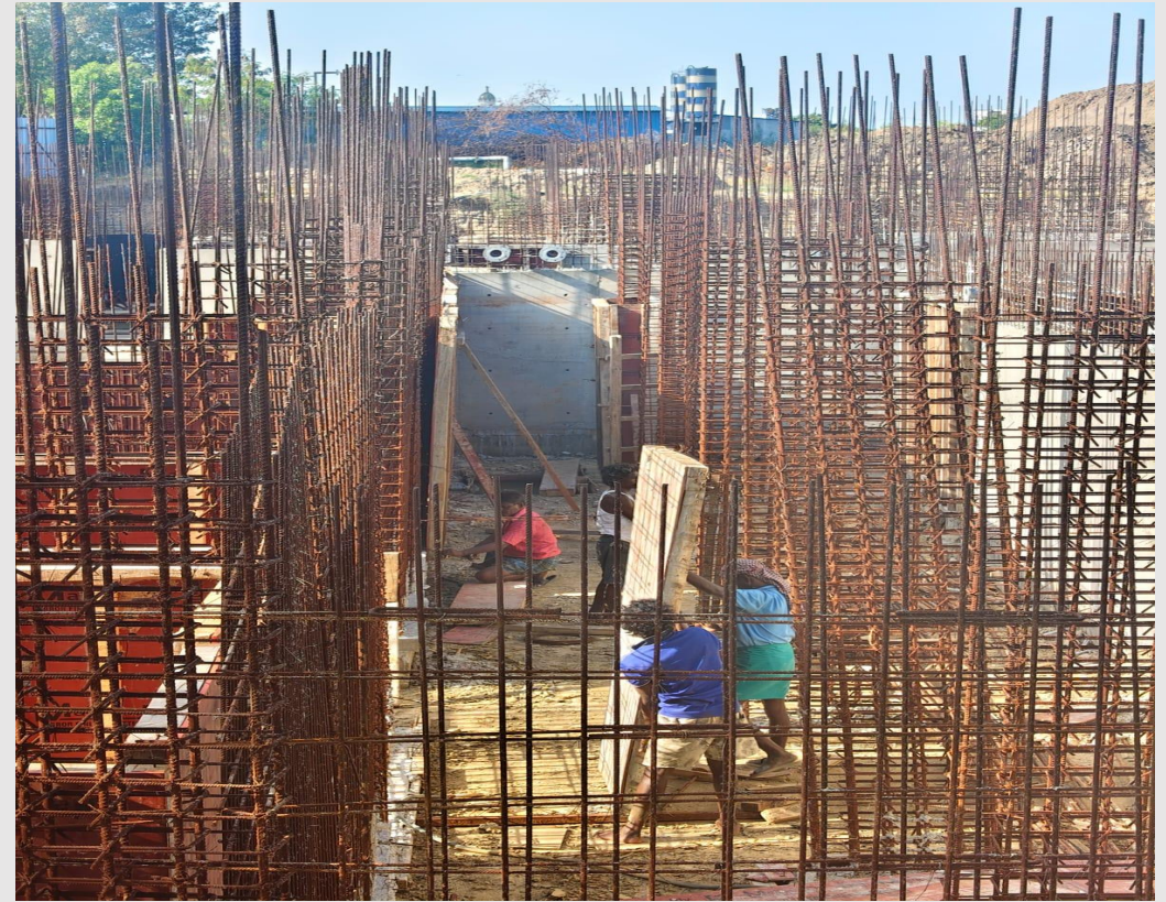
U G sump pump room shuttering works in progress
