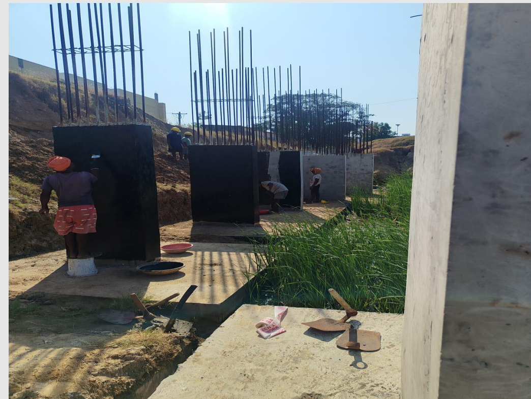
Waterproof coating work in progress
