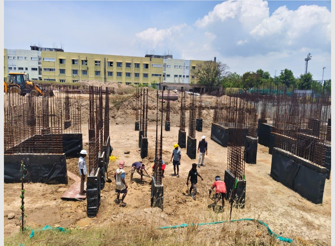
Soil leveling & reinforcement work
