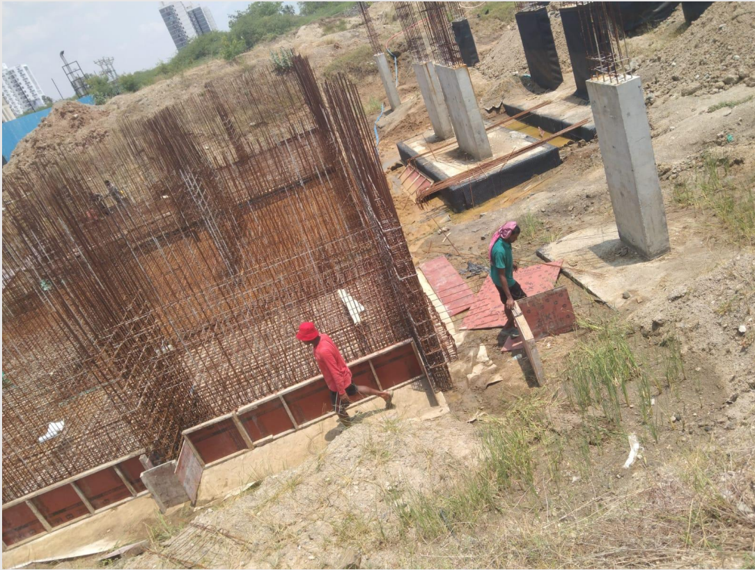
UG Sump shuttering in progress
