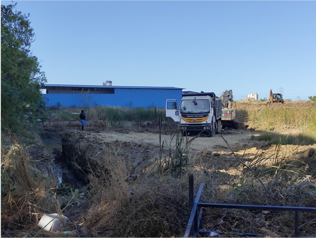
Excavation work in progress
