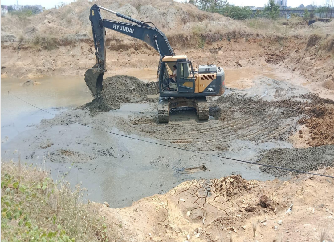
Sump area excavation work in progress
