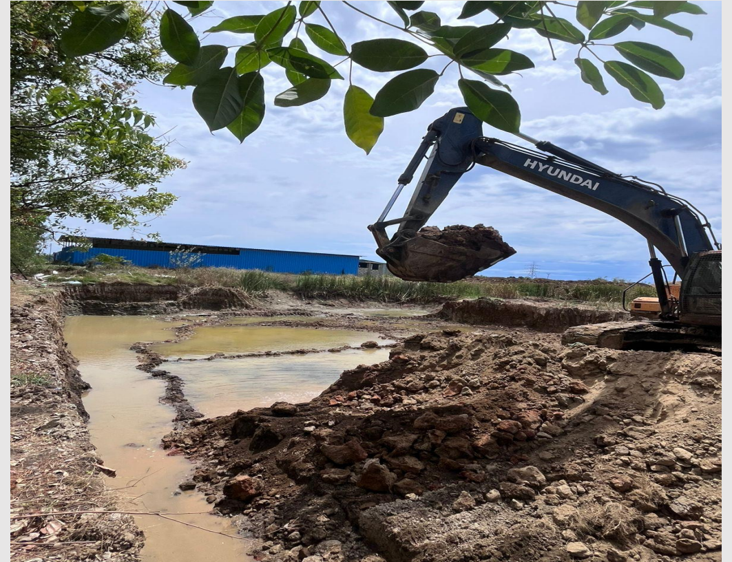
Excavation along with dewatering work in progress
