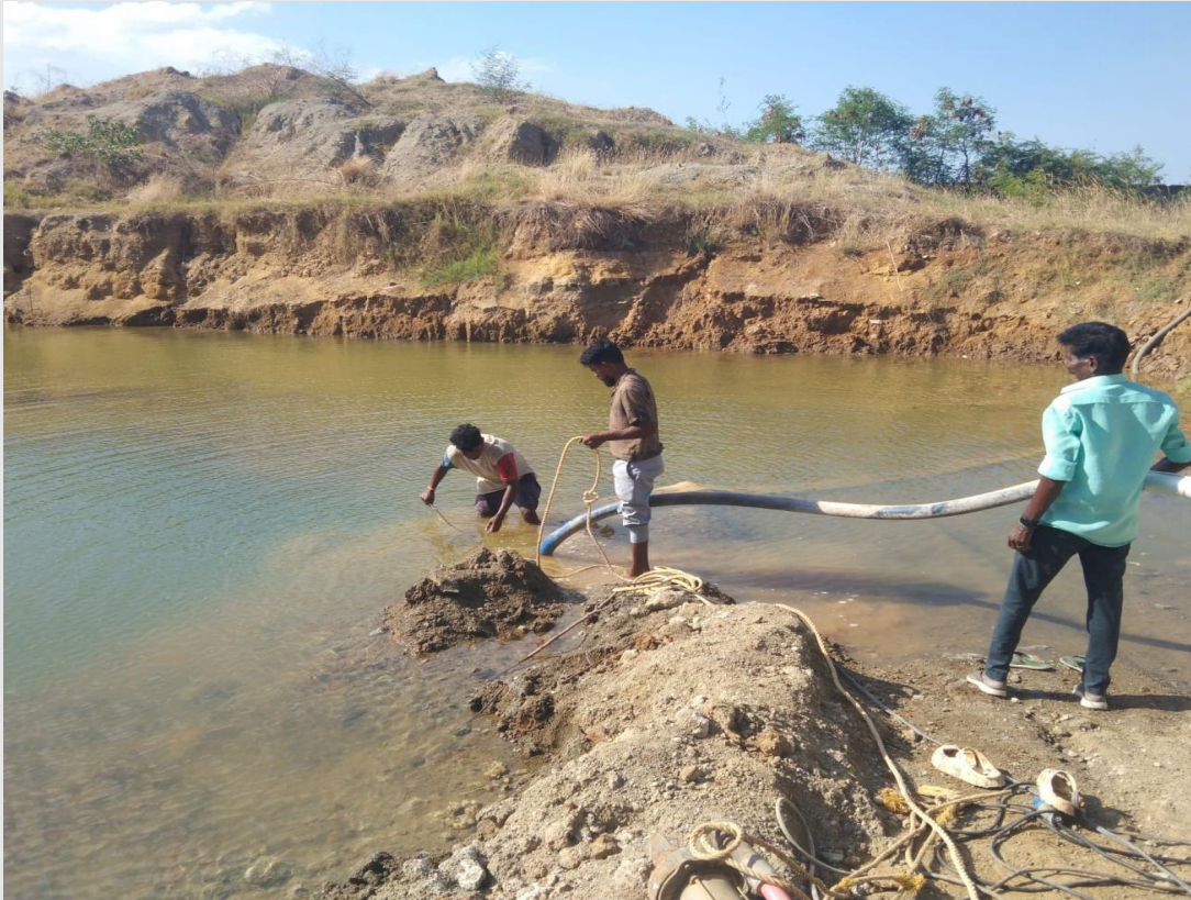
Dewatering work in progress
