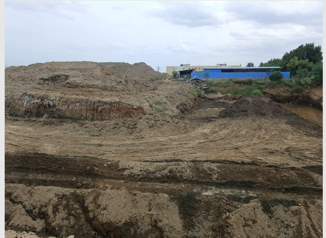
Excavation work in progress
