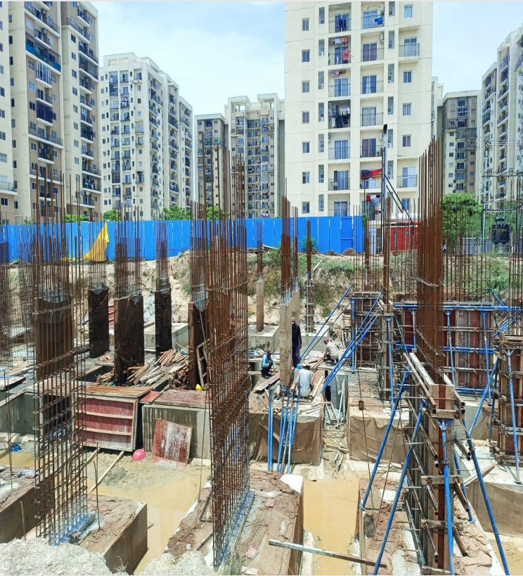
Footing and column reinforcement and shuttering works in progress. 7nos column concrete planned
