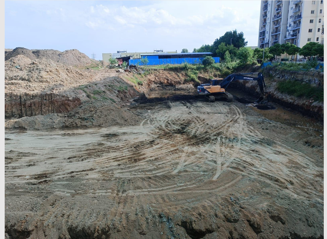
Excavation work in progress
