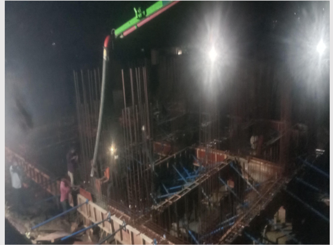
plinth beam concrete work
