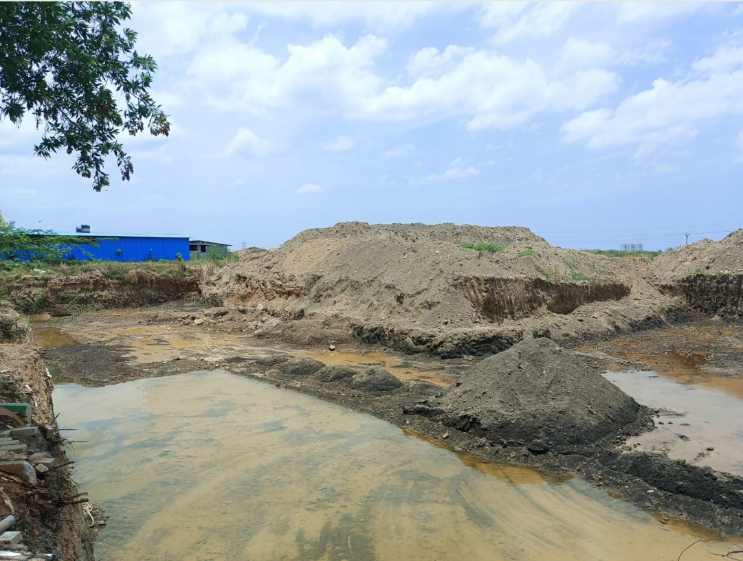
footing PCC Preparation works in progress
