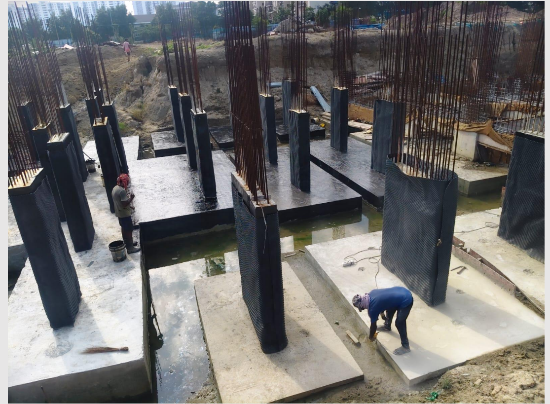
Waterproofing coating preparation work in progress
