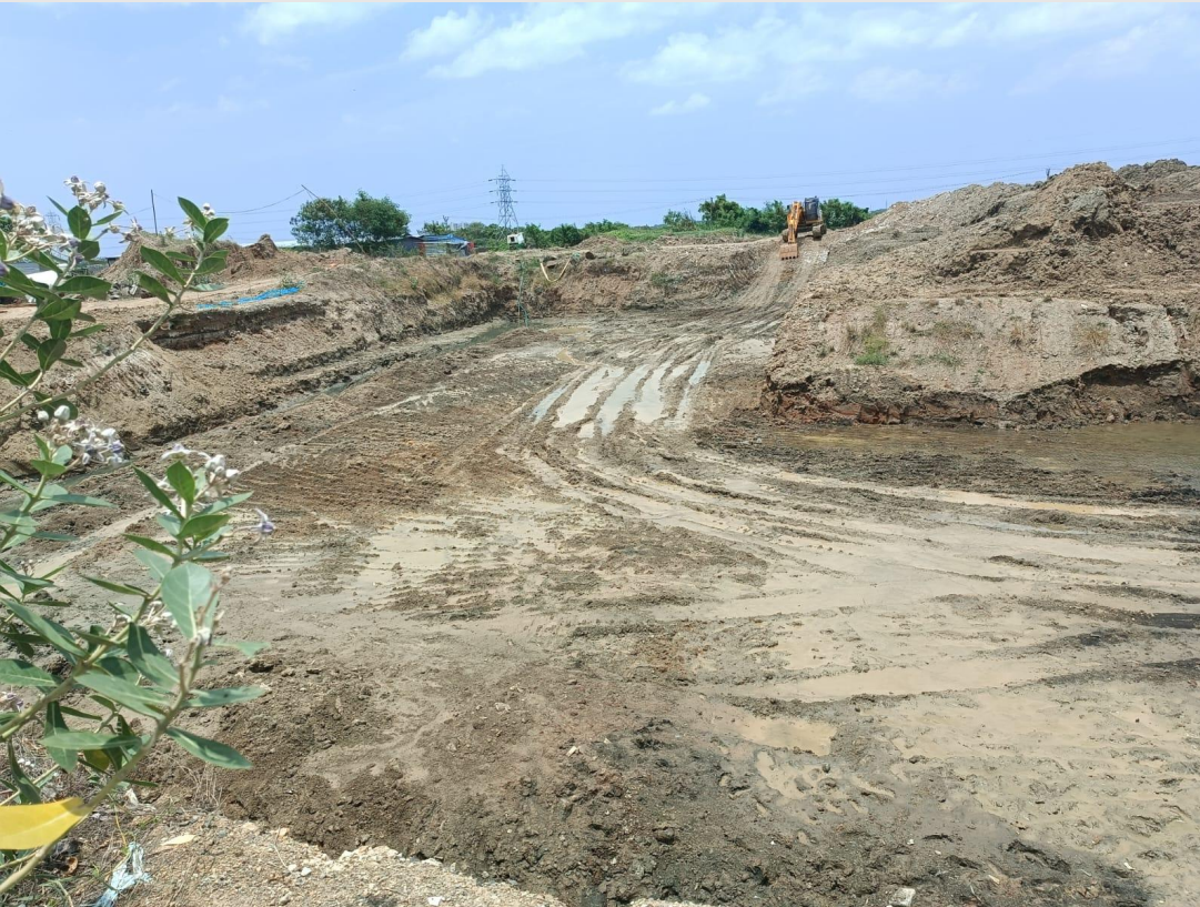
Excavation 2.5m depth completed
