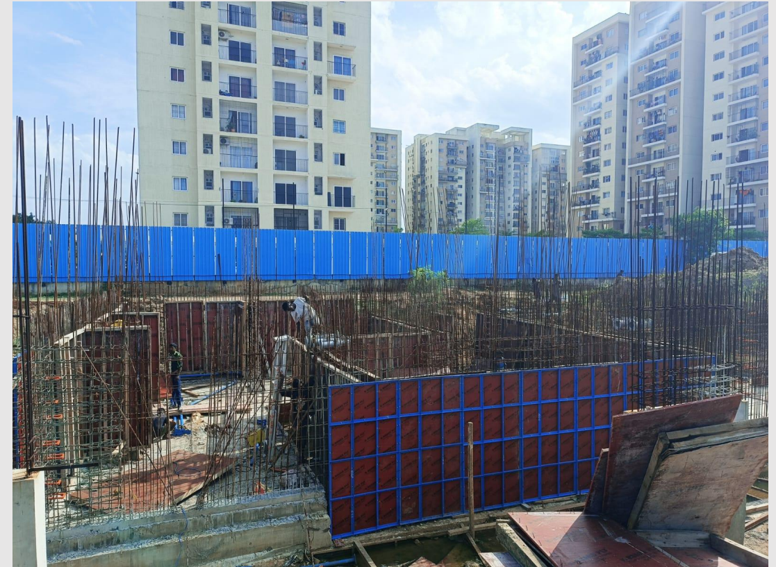
UG Sump wall shuttering work and plinth beam PCC Preparation work, stilt floor column reinforcement work
