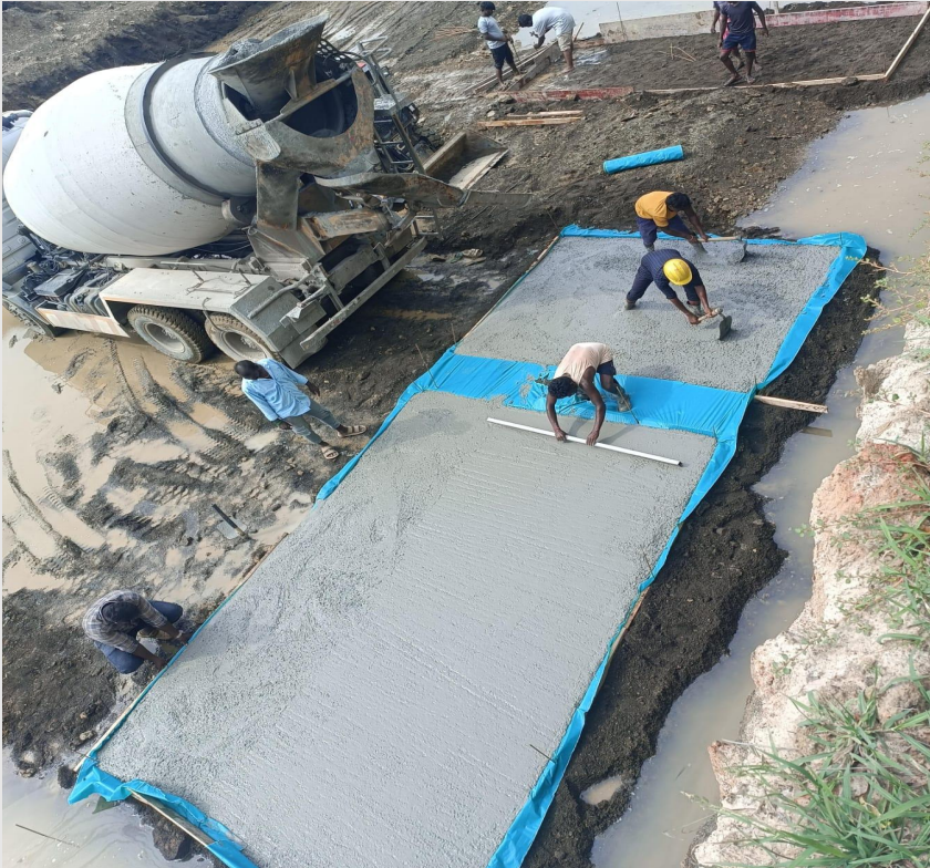
Footing PCC work in progress
