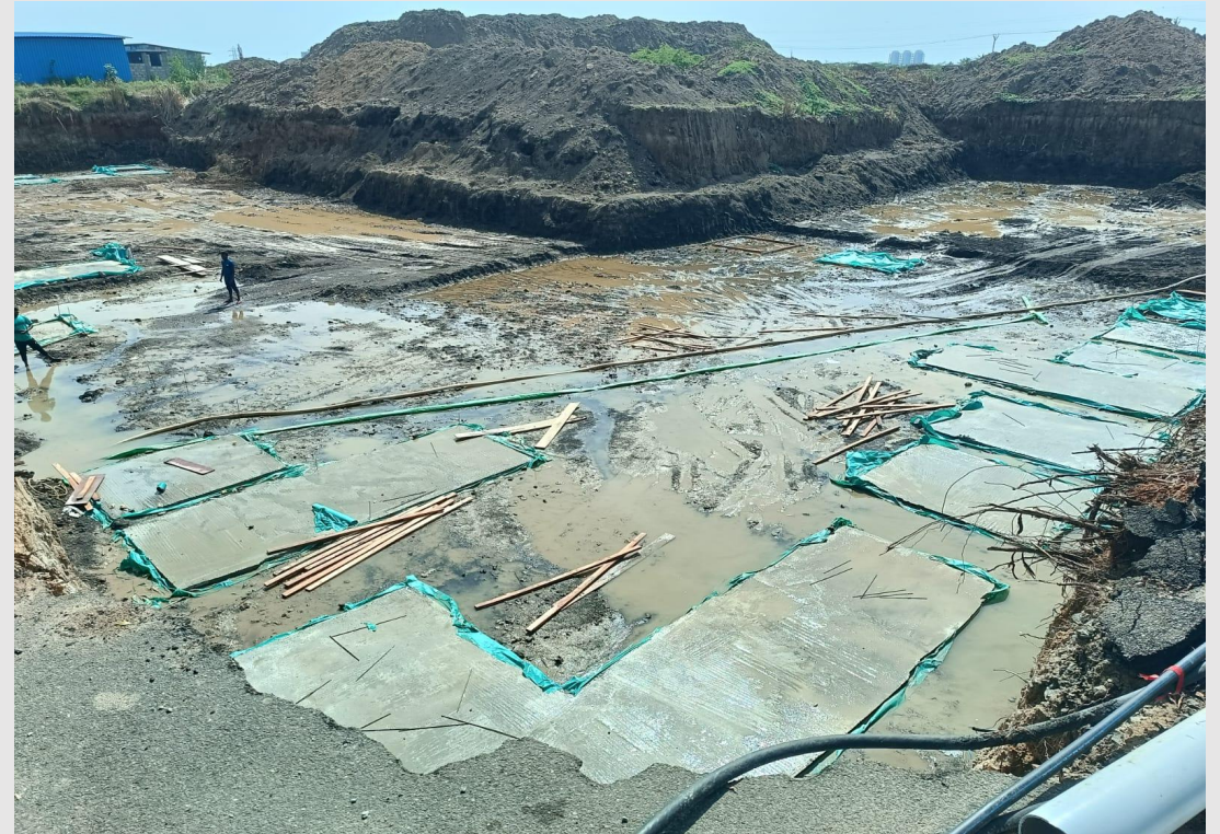
Footing PCC Works in progress
