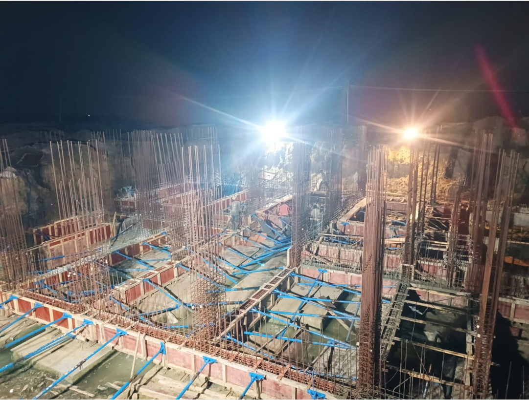
Plinth beam shuttering work
