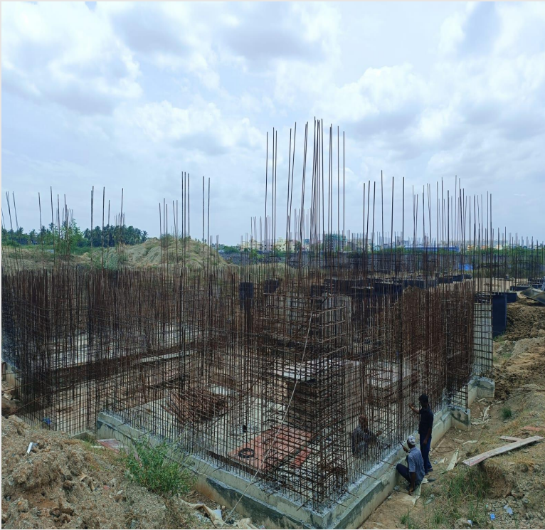
UG wall reinforcement distribution works in progress. wall shuttering board making works in progress
