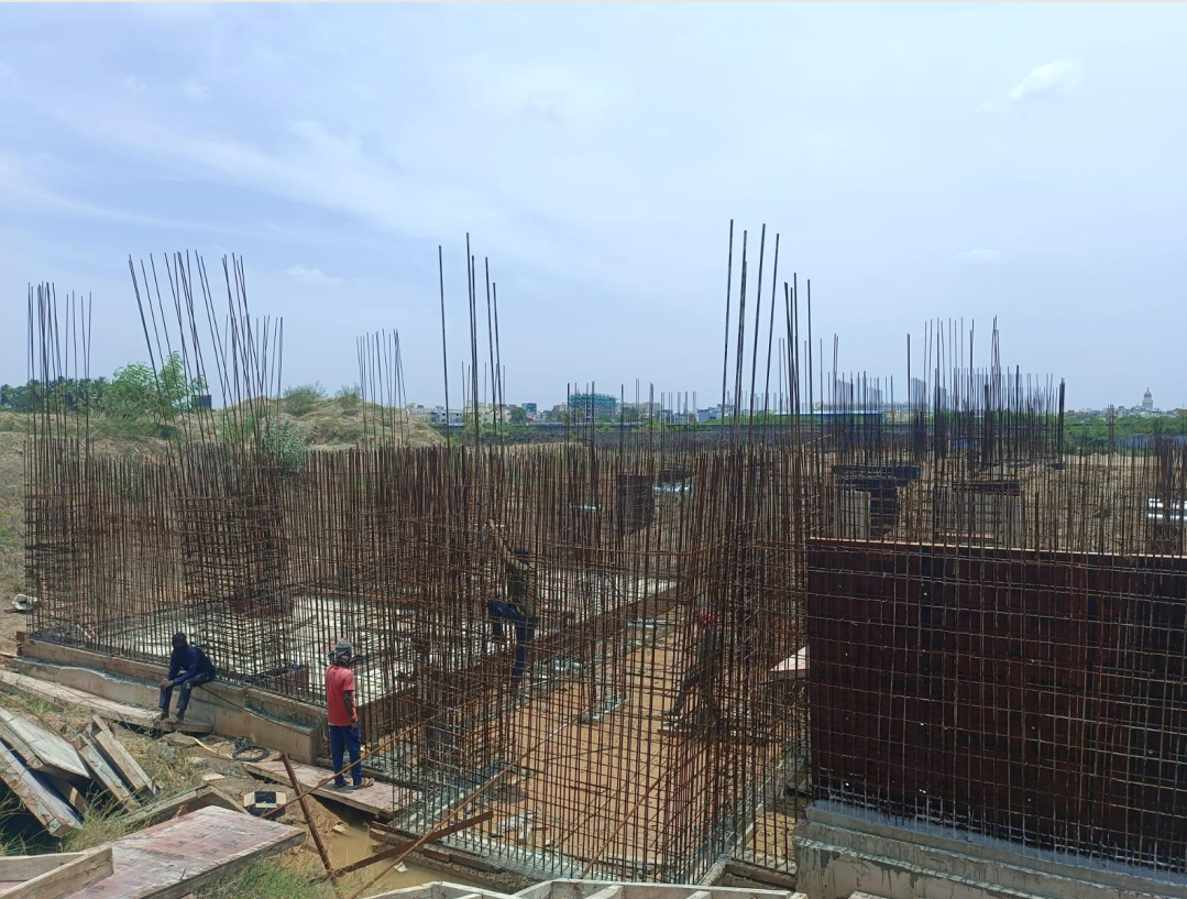
Ug sump wall shuttering works and plinth beam. PCC Soil leveling works
