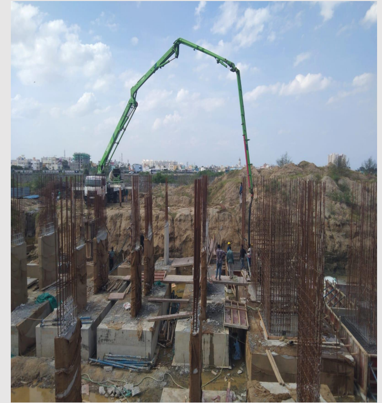
Footing and column reinforcement work and shuttering work in progress. 4nos footing concrete work in progress
