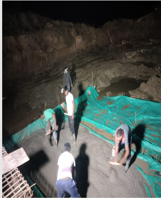
footing PCC concrete work
