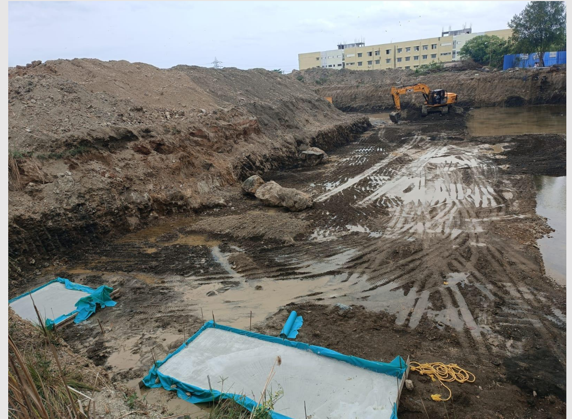
Footing PCC Preparation works in progress
