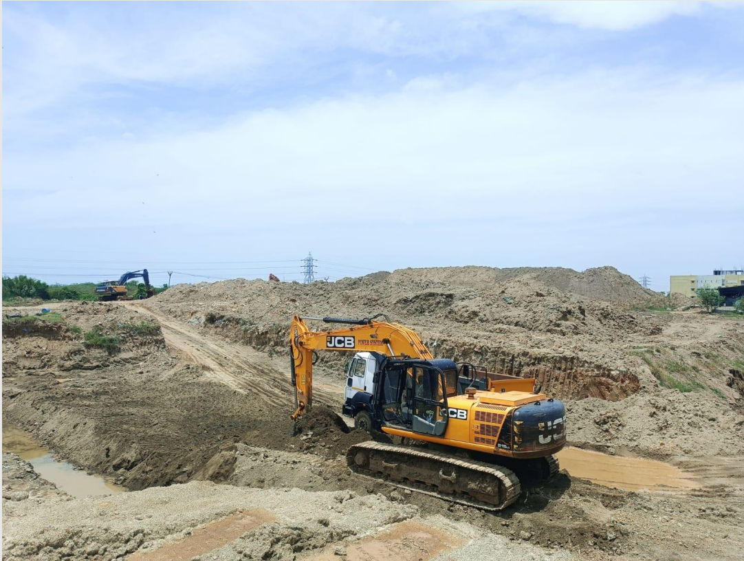
Excavation works in progress
