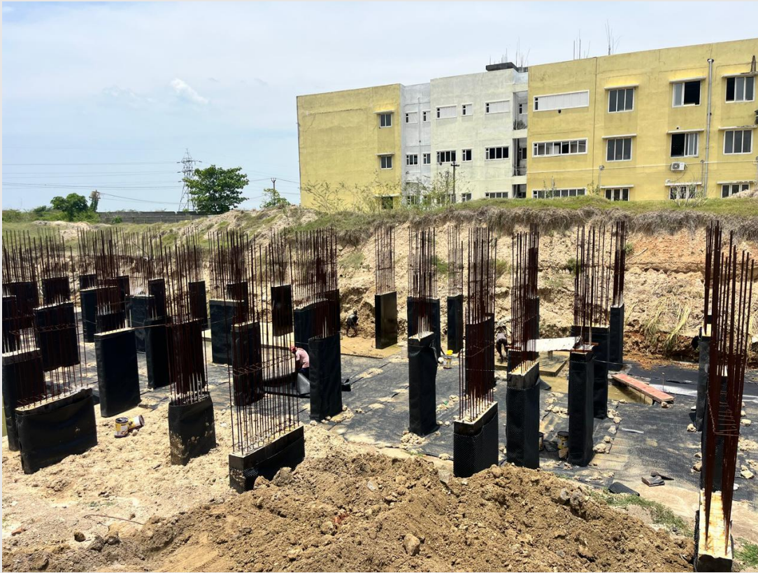
waterproofing works in footing and column in progress. backfilling works in progress
